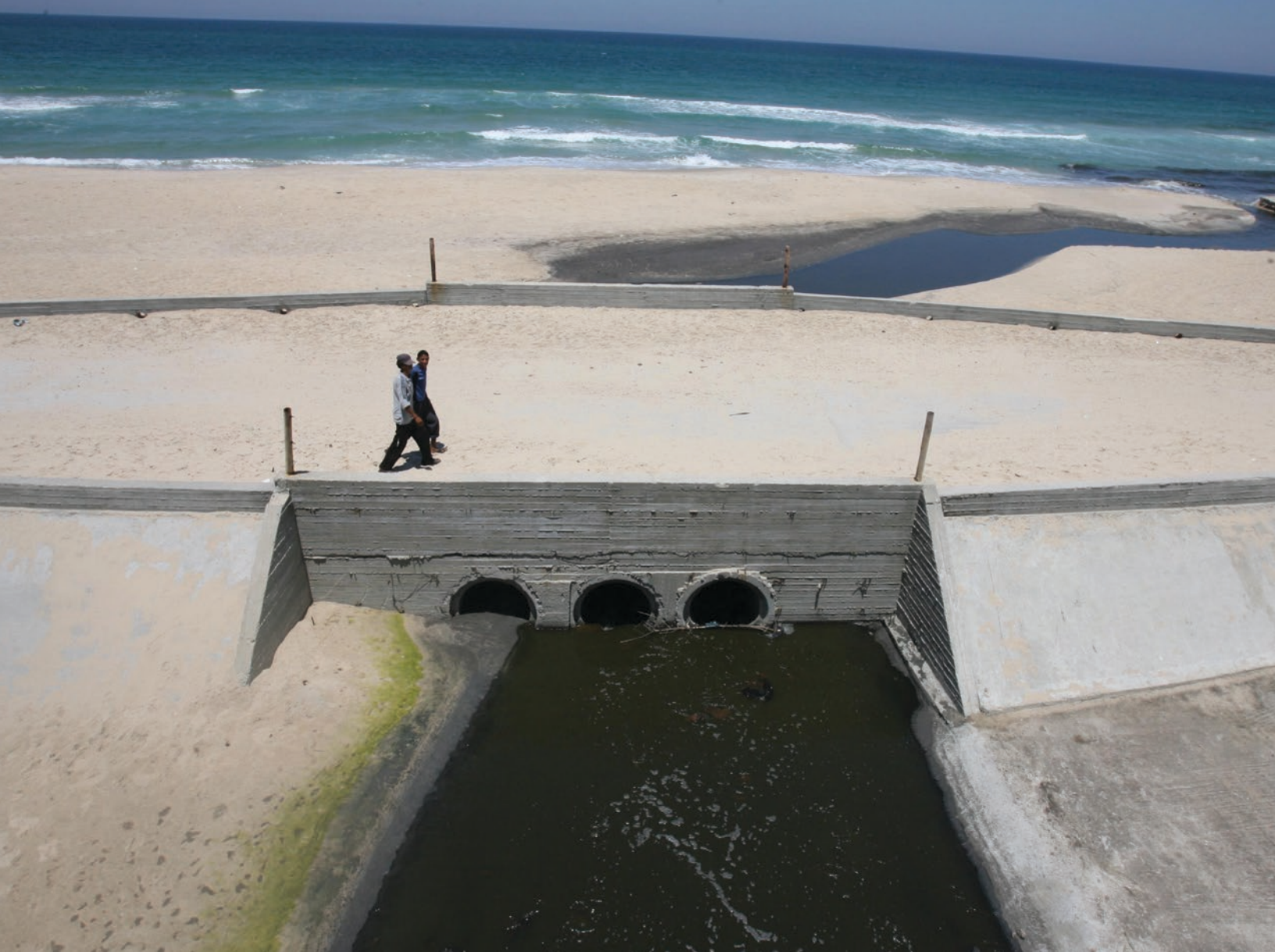
Raw wastewater flows into the Mediterranean Sea near Deir Balah, Middle Area, Gaza Strip. © ICRC.
