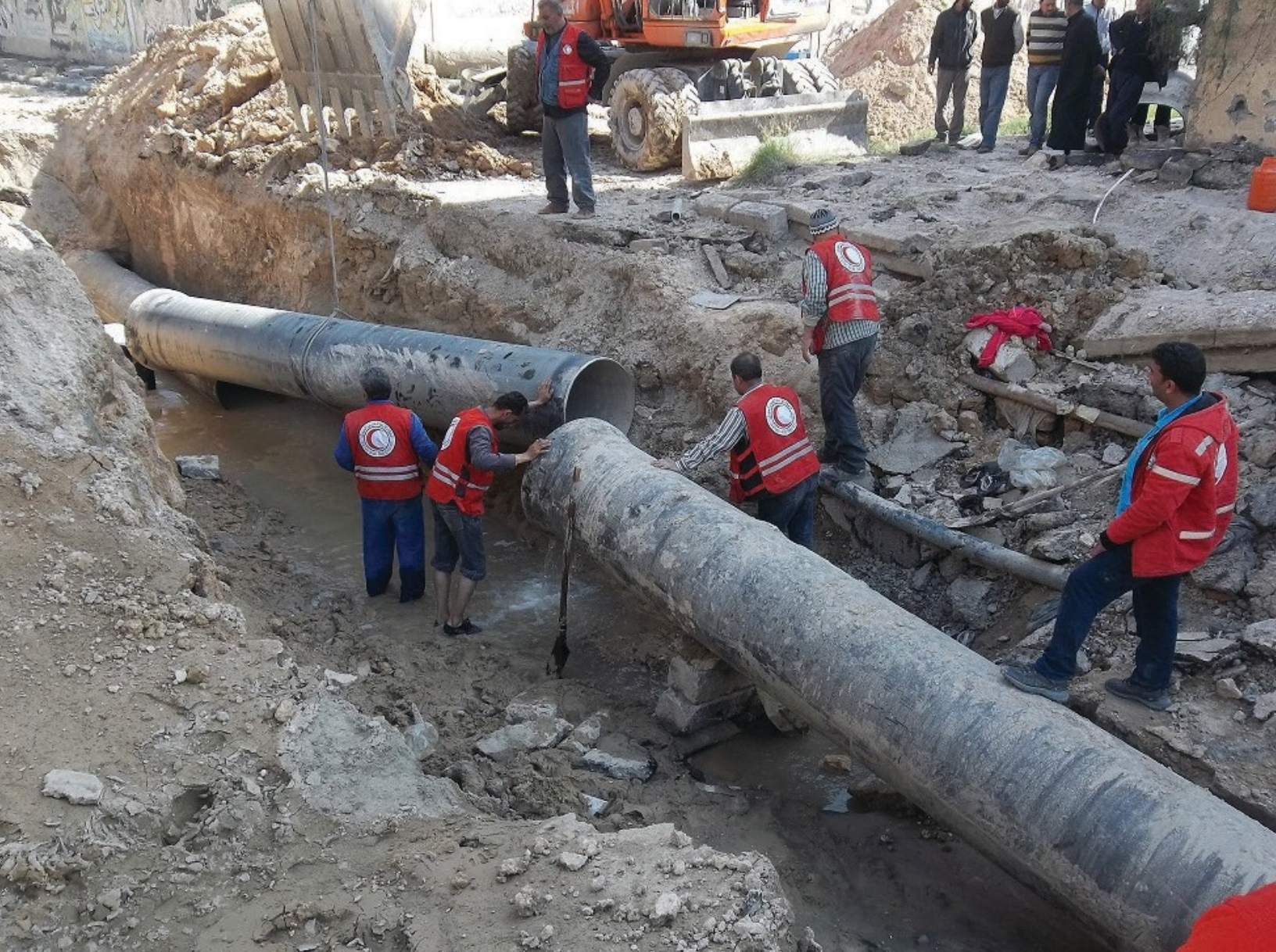
Maintenance of water pipeline (700 mm) in Deir Ezzor city in 2014. This water pipeline from Al Basel pumping station feeds many neighborhoods in the city (approximately 30,000 beneficiaries). The pipeline was severely damaged due to the hostilities in the area. These emergency repair works were carried out on the frontline after a ceasefire was agreed. © M. Al Ali/SARC.
