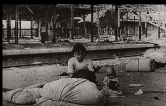
China, 1937. Sino-Japanese war, 1937-1938. Bomb damage at Shanghai's southern train station.
