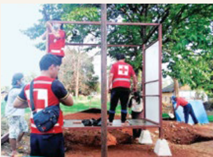
Construction of temporary latrines were installed at quarantine centres in Lashio to help prevent the spread of COVID-19.
