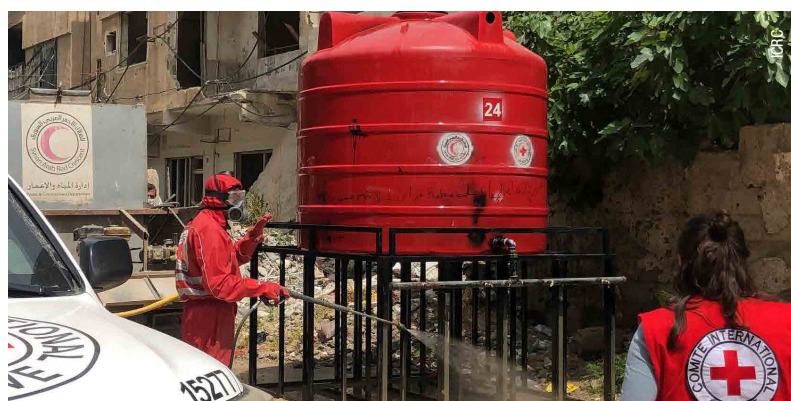
Syria, Eastern Ghouta. On a daily basis, the Syrian Arab Red Crescent and the ICRC fill and sterilize one of 225 water tanks providing drinking water to some 200,000 people.
