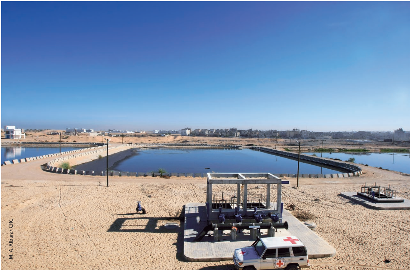
Part of a large-scale water-treatment system in Gaza.
