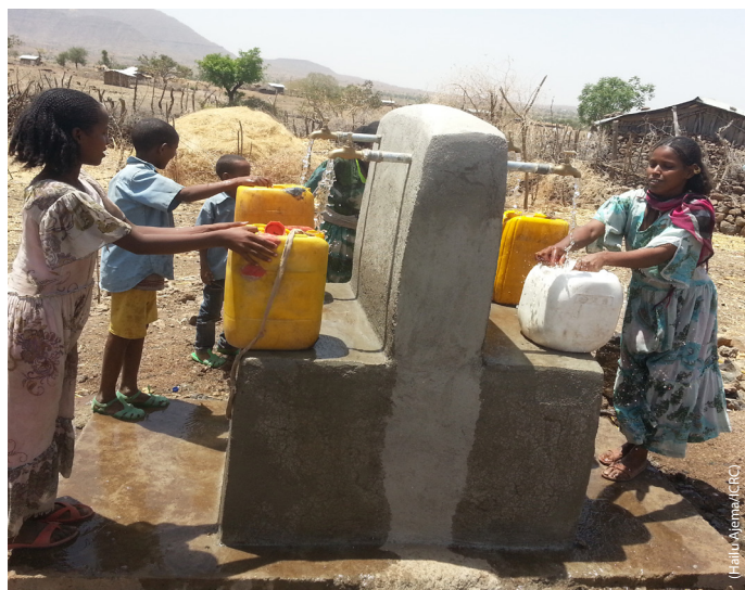
A water facility built to improve access to water for drought-affected communities in Kaftahumera, Tigray, by the ICRC, 2015.
